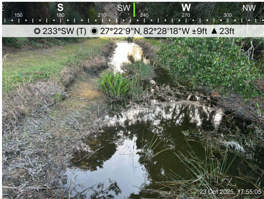
Photo 10 – Representative view of stormwater ditches observed onsite.
