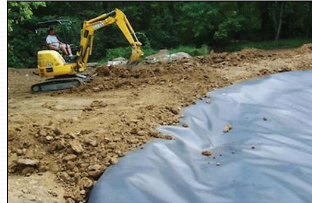
Geotube reinforced banks ($70-$100 per linear foot)
