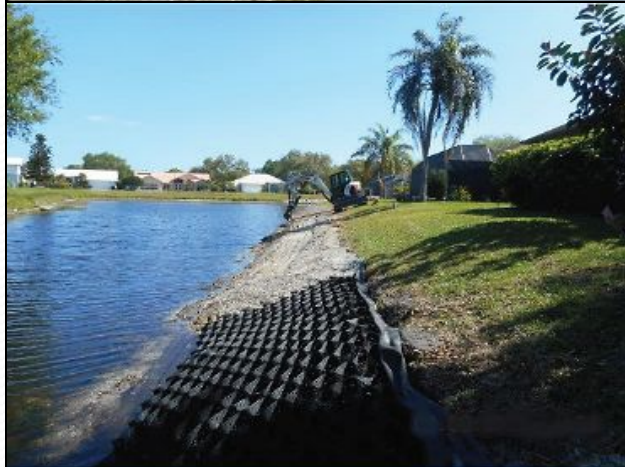
Geoweb reinforced banks ($100-$150 per linear foot)
